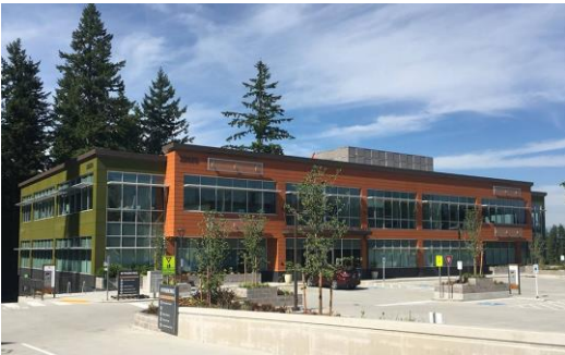
Sammamish Village Medical Pavilion
