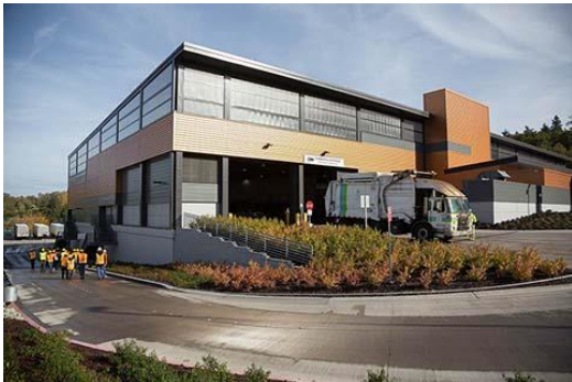
Factoria Transfer Station
