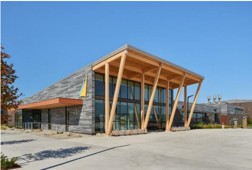
Oak Harbor Clean Water Facility
