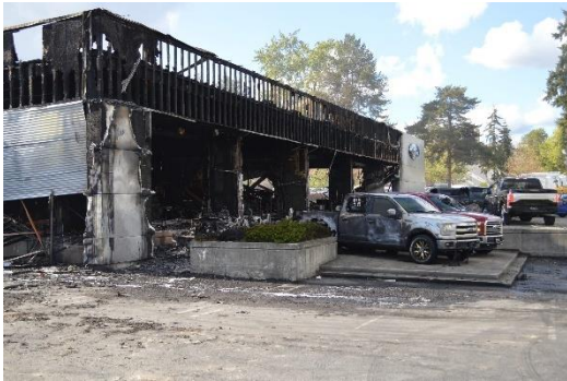
Ford of Bellevue Fire Restoration
