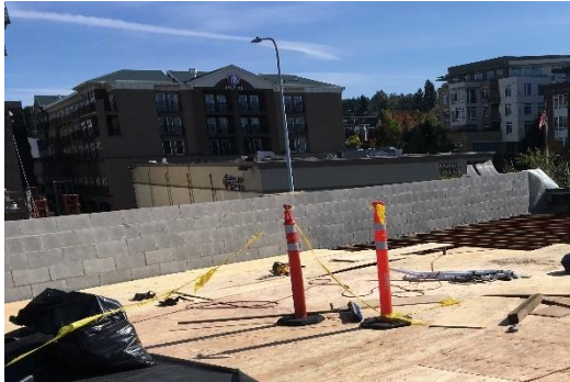
Park Lane Roof Shoring
