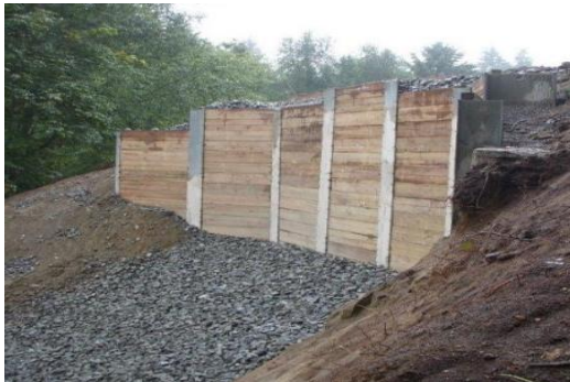
Heronfield Shoring Stabilization
